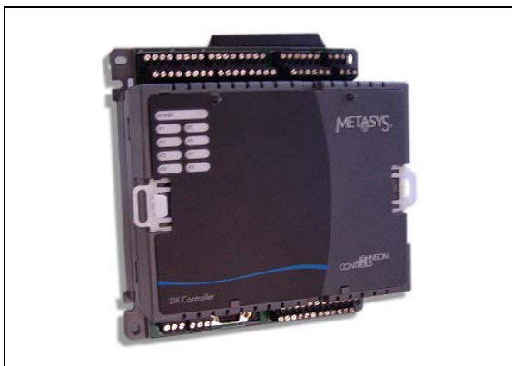
Figure 6: DX-9200 Controller – Black Box – on Panel Mounting Base
